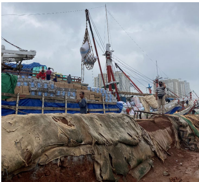
Figure7 : The condition of the quay and the process of cargo handling.
