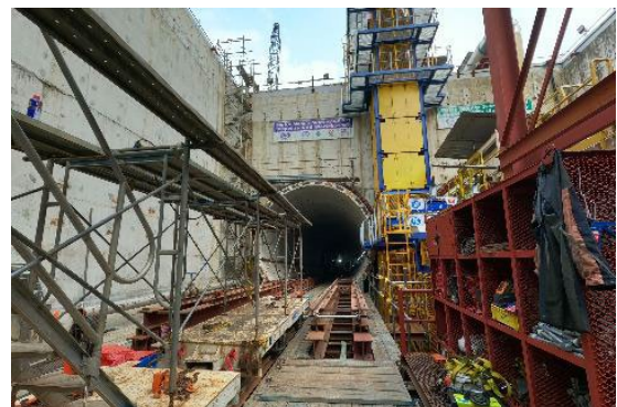
Picture-6 Inside the TBM Launch Shaft
