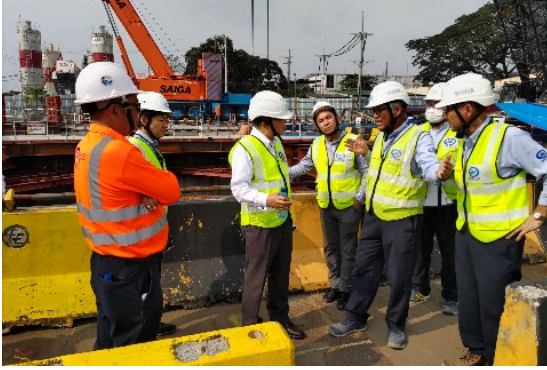
Picture-9 Scene of the Construction Site Visit
