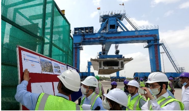
Picture-5 Hoisting work by a straddle carrier
