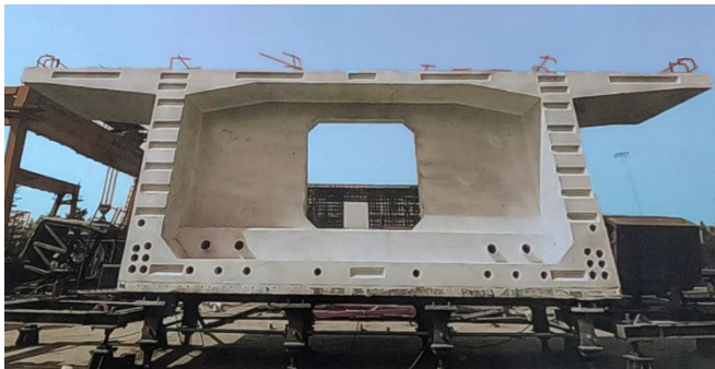
Picture-1 Cross section of a segmental girder
