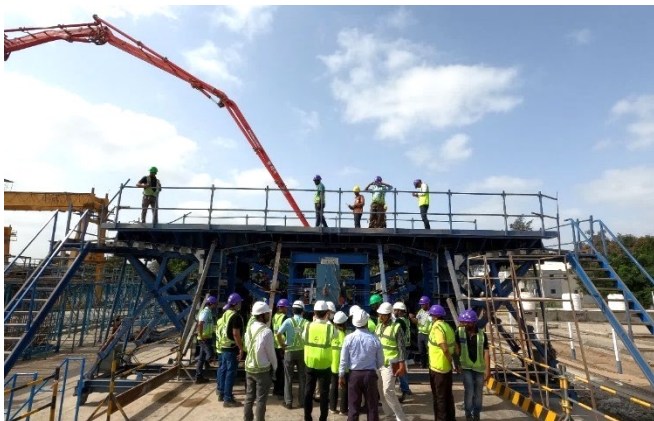
Picture-2 Casting work
