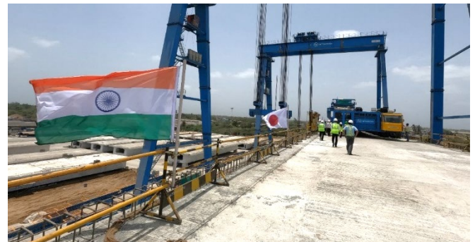
Picture-9 National flags on the viaduct
