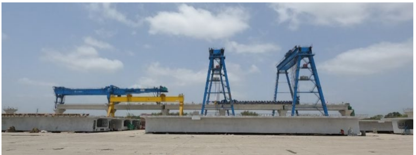
Picture-7 Overview of the casting and erection yard
