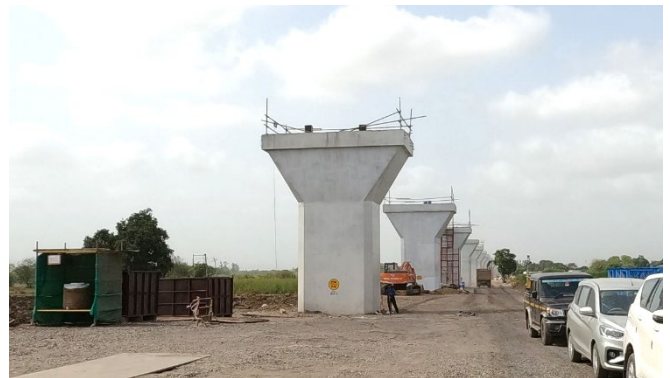
Picture-4 Completed piers
