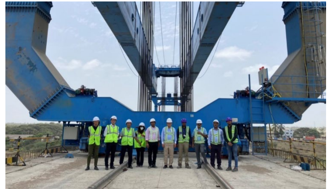
Picture-8 A launching gantry on the viaduct
