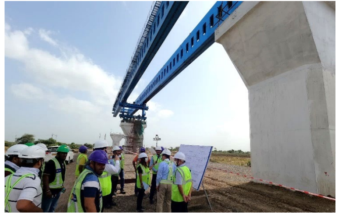
Picture-3 Overhead launching gantry
