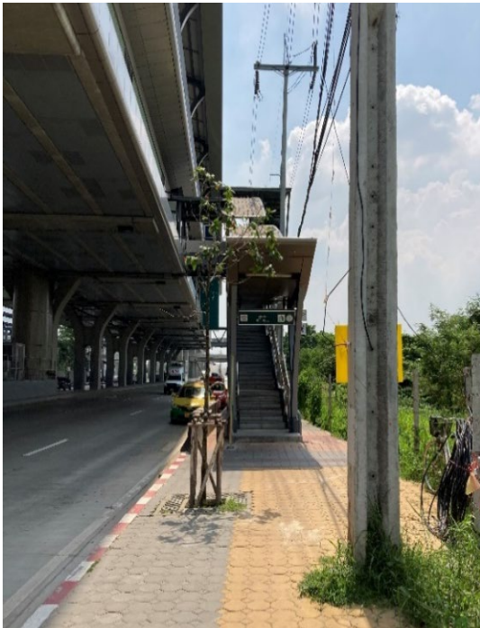
Photo-7: Stairs on the sidewalk
