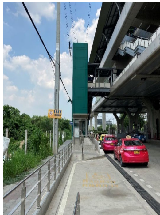
Photo-8: Elevator on the sidewalk
