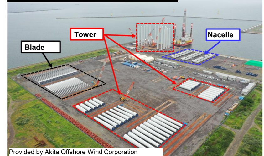
Placement of windmills at Noshiro Port (completed in Sep. 2022)
