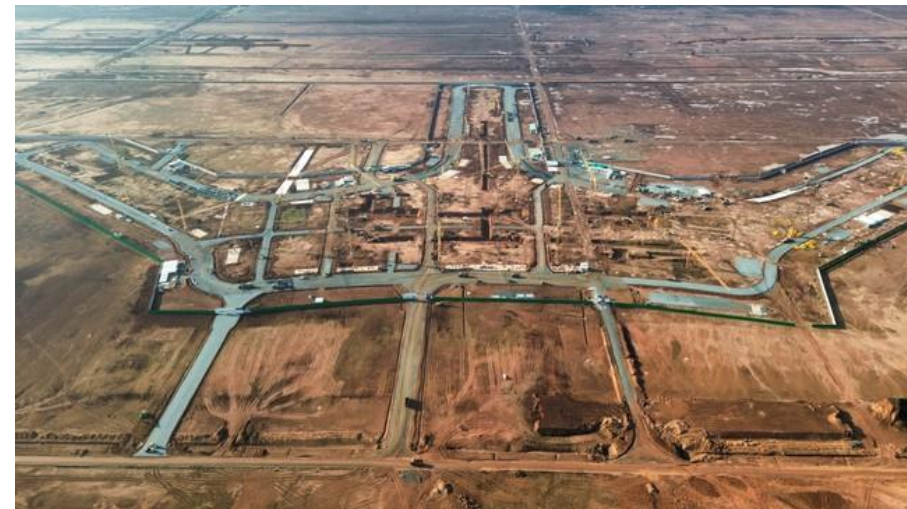
Long Thanh International Airport
